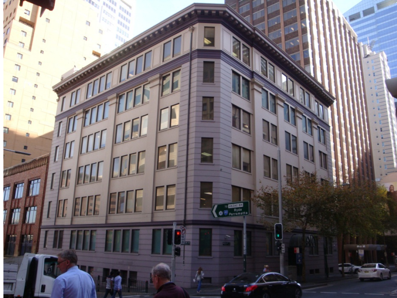
Figure 1: 453 Kent Street Sydney as at May 2014
