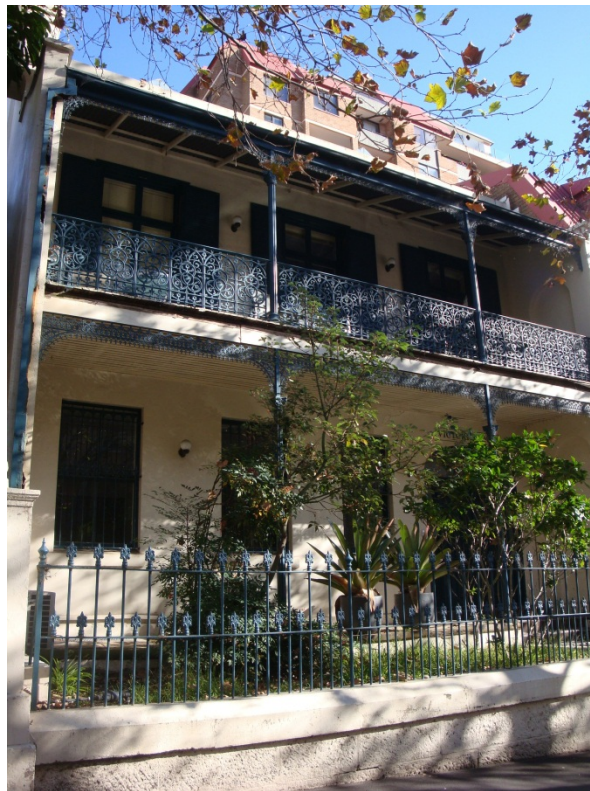
Figure 3: 97 Victoria Street Potts Point at May 2014
