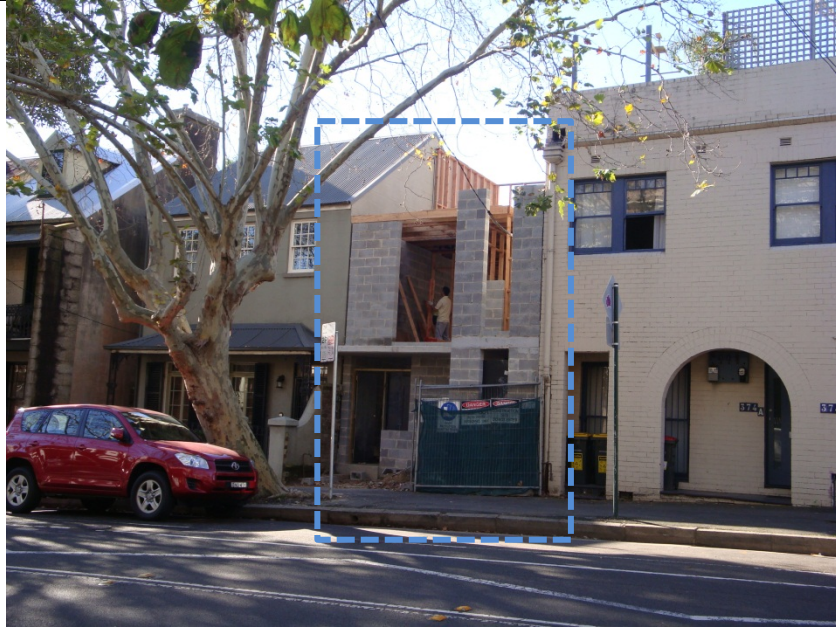
Figure 2: 372 Riley Street Surry Hills as at June 2014
