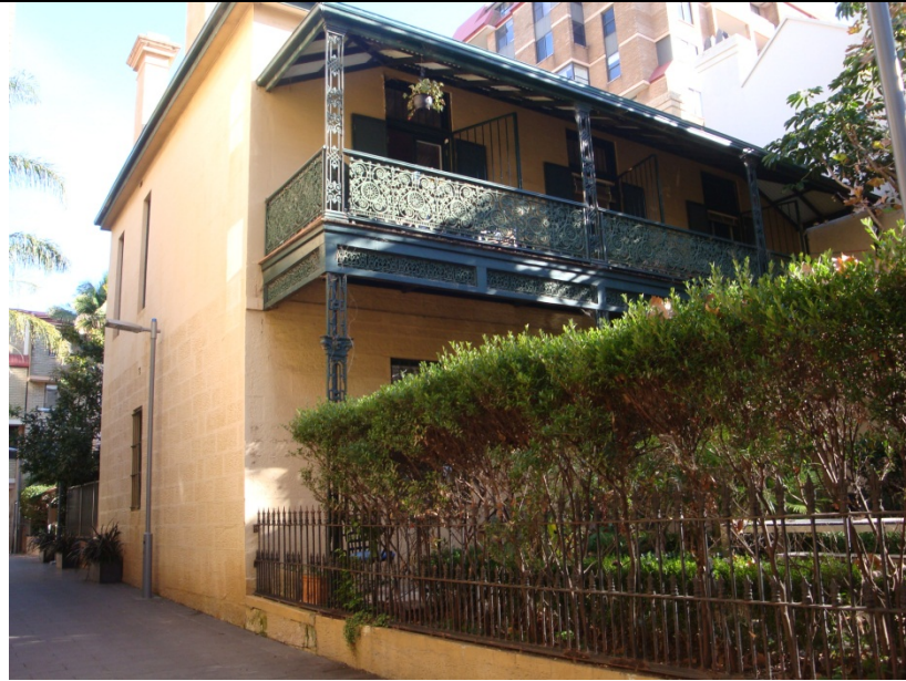
Figure 4: 99 Victoria Street Potts Point at May 2014
