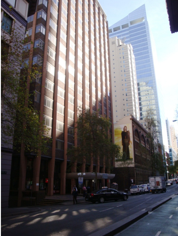
Figure 3: 443-451 Kent Street Sydney as at May 2014
