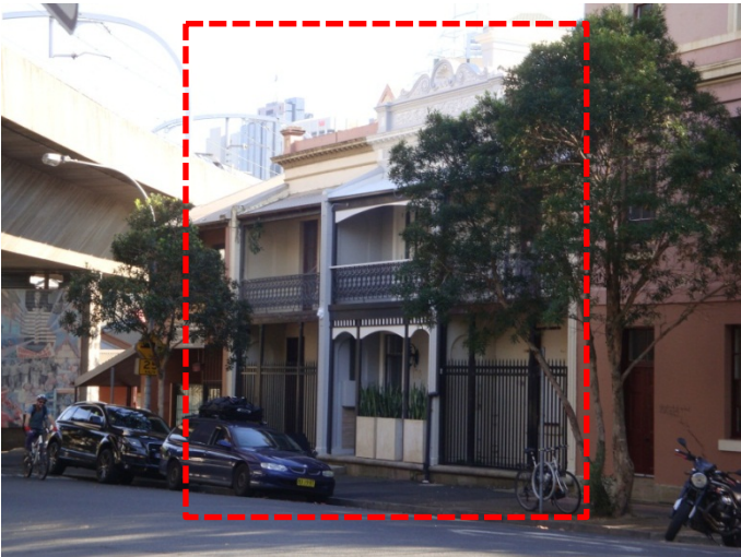
Figure 1: 168, 170 and 172 Cathedral Street, Woolloomooloo
