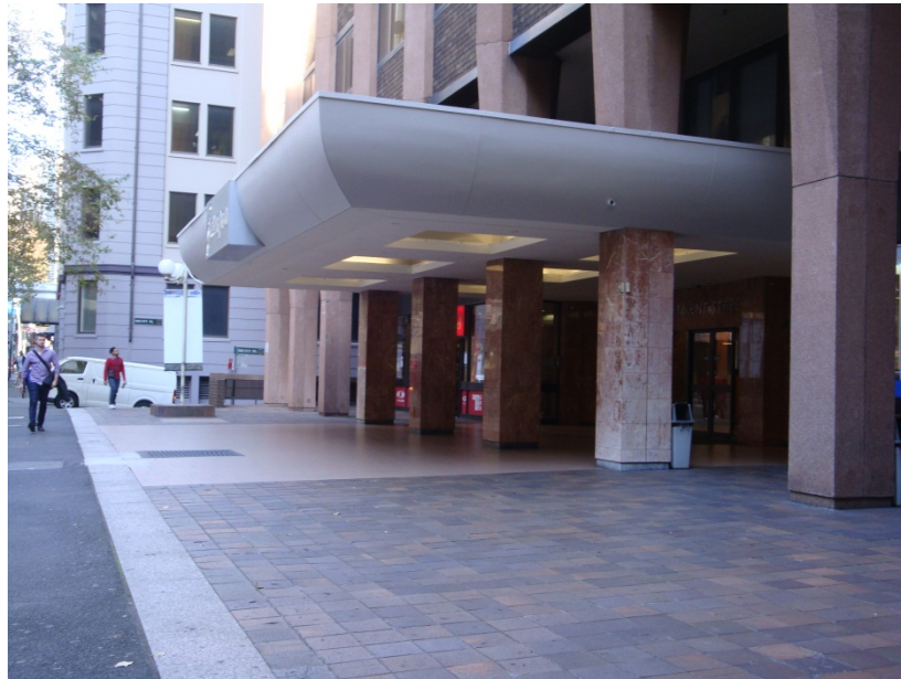
Figure 4: 443-451 Kent Street Sydney open space at street level as at May 2014
