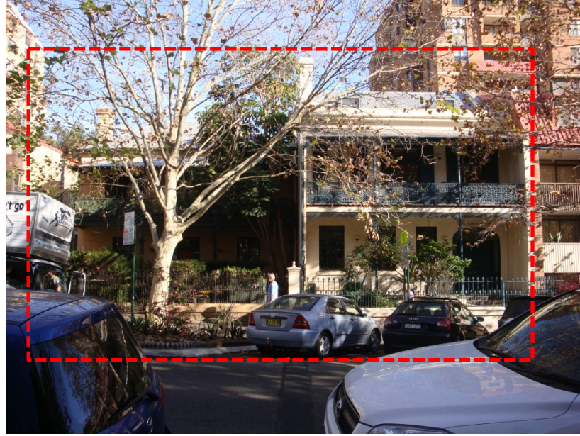
Figure 2: 97 and 99 Victoria Street Potts Point at May 2014
